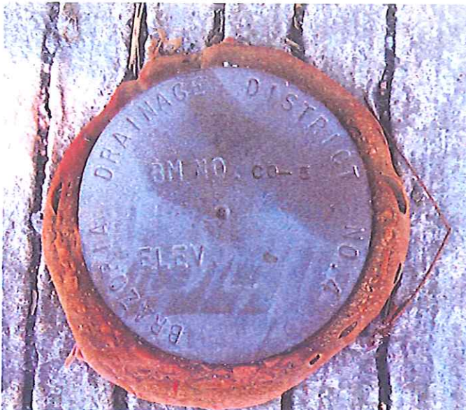
Photo – Station Detail
