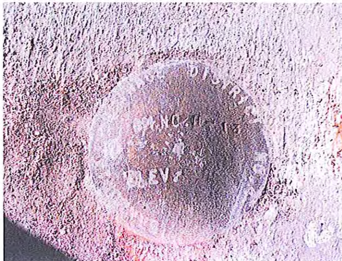
Photo – Station Detail
