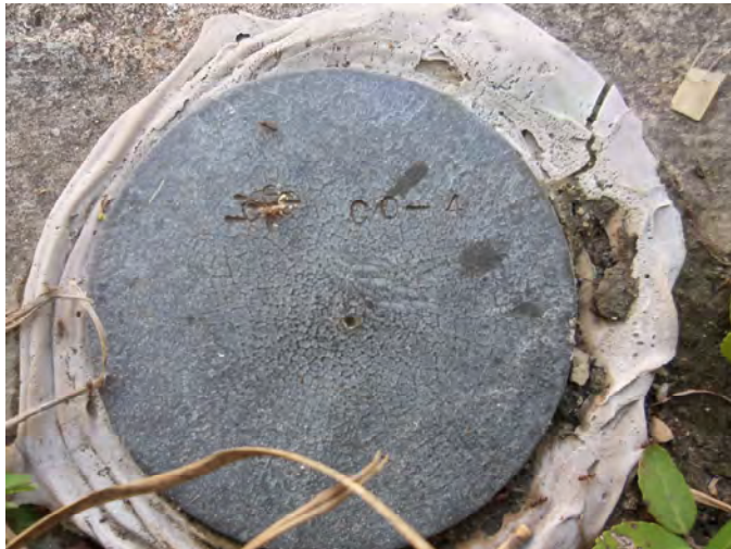
Photo – Station Detail
