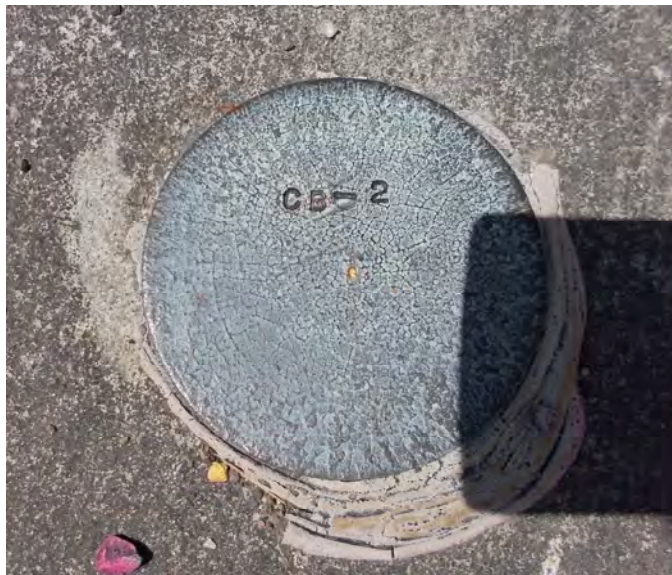
Photo – Station Detail
