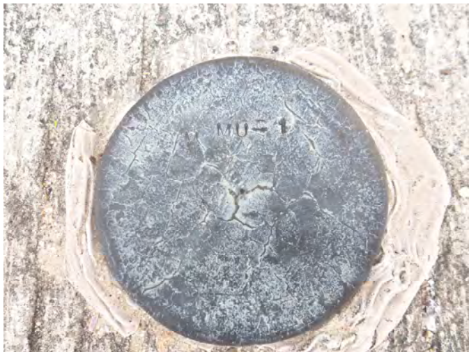
Photo – Station Detail
