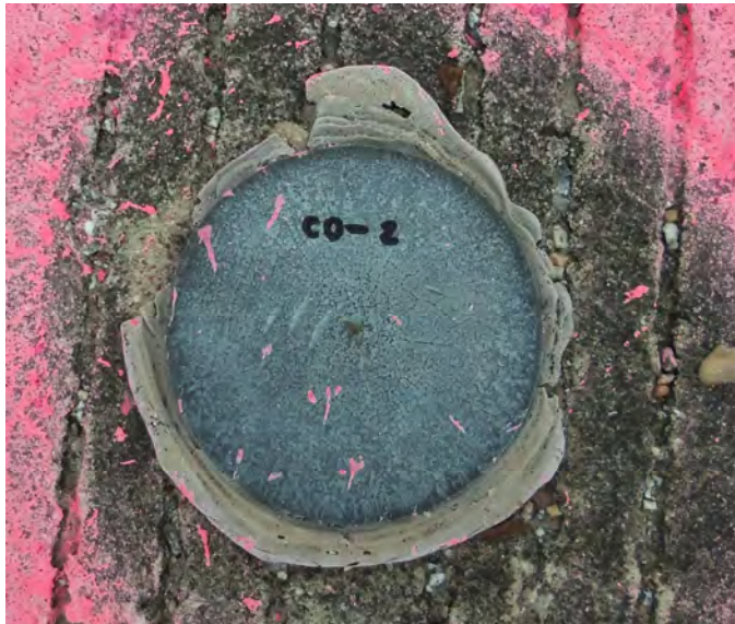
Photo – Station Detail
