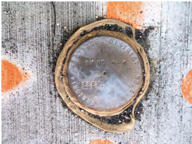
Photo – Station Detail
