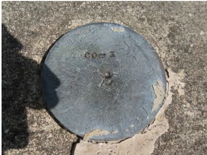
Photo – Station Detail
