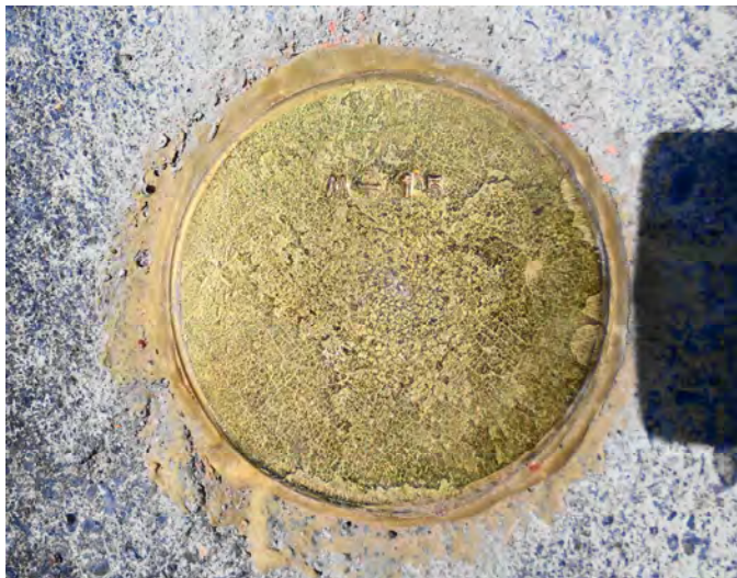
Photo – Station Detail
