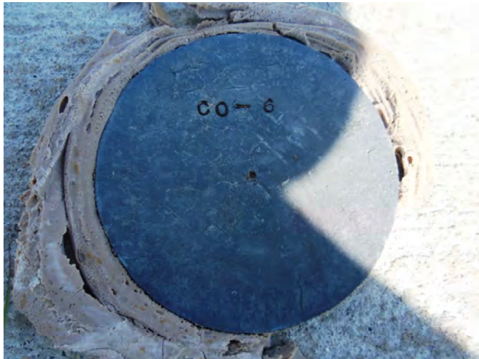
Photo – Station Detail
